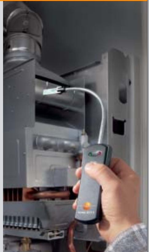
Establishes if flue gases have been drawn off completely from the burner
