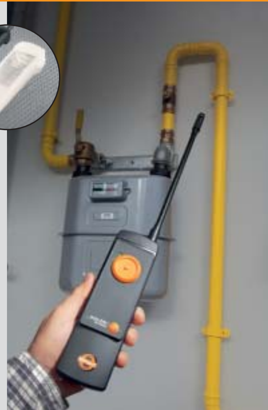
Checks for leaks in domestic gas pipes
