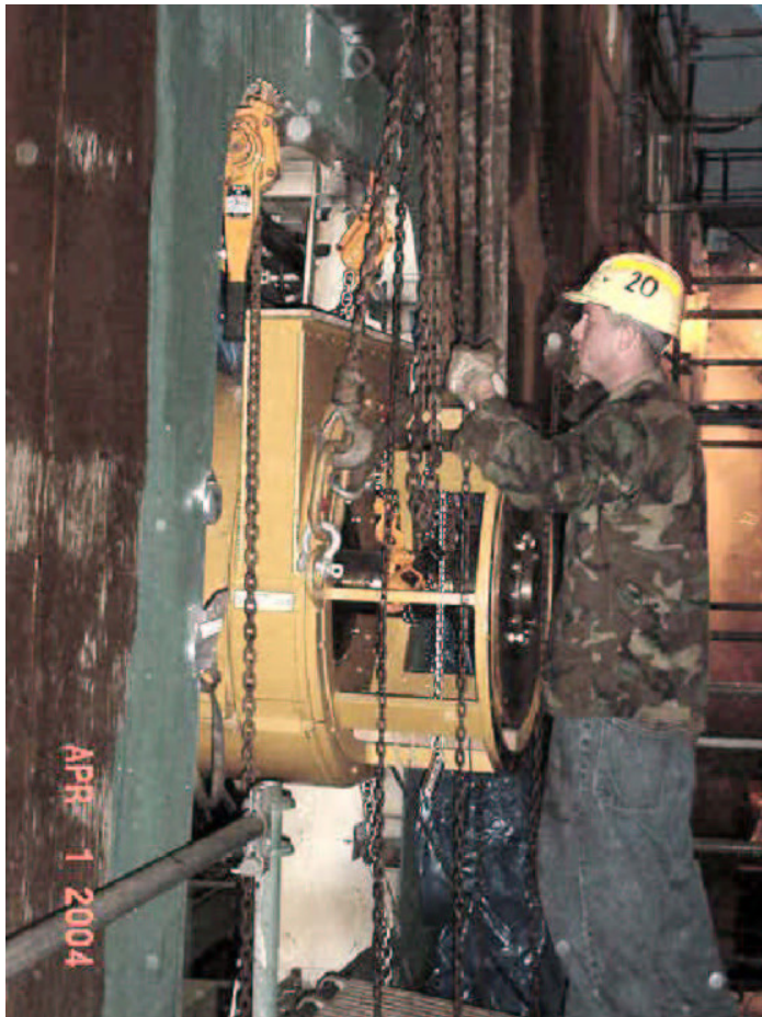
Figure 7. Generator Removal
