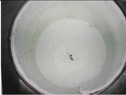
Figure 5. Overlapping vacuum formed insulation
