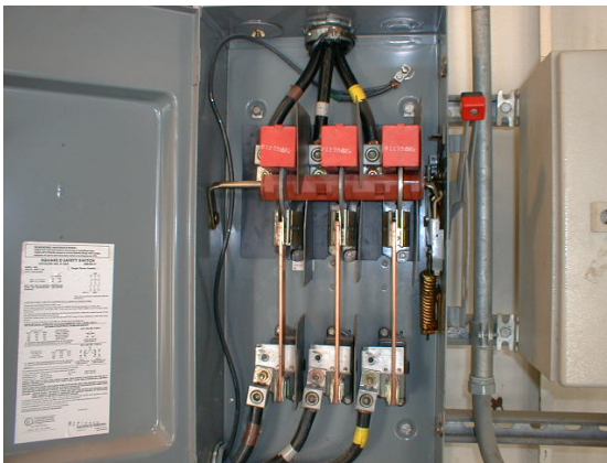
Figure 9: Visual and thermal images of a faulty disconnect switch
