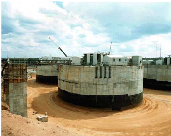
Figure 2. Waste tank construction
